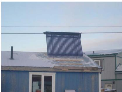
King Span solar evacuated tube (30) (@ 68degrees)
