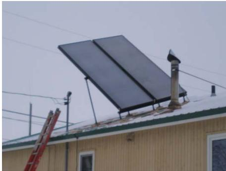
Gobi 410 flat plate (2). Mounting brackets rated to withstand 100mph winds.
