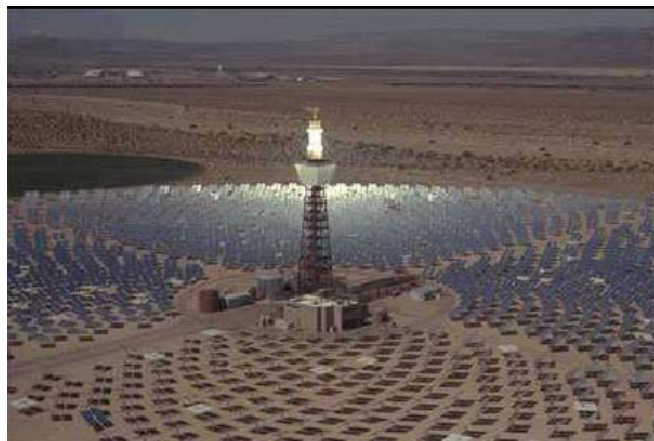
Fig. 5 – Aerial view of Solar Two
