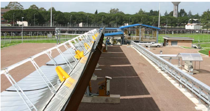
Fig. 10 – PCS test field at ENEA - Casaccia (Rome)
