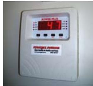
A controller is required on pumped systems to turn the pump on when sufficient heat is available at the collector to heat the water, and off when there is not.
