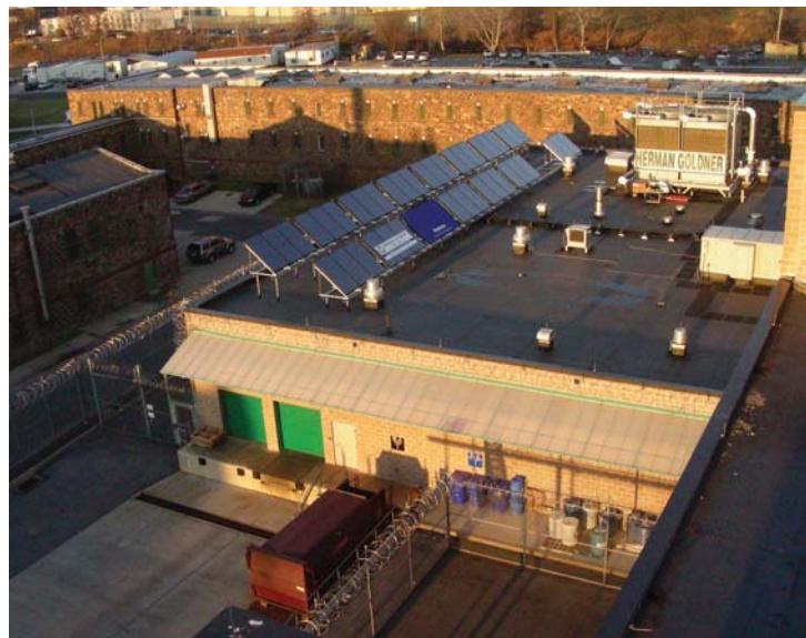
Aerial view of roof-top solar array at Riverside Correctional Facility. The 80 year-old brownstone House of Correction is immediately behind, and the Detention House is visible in the distance.
