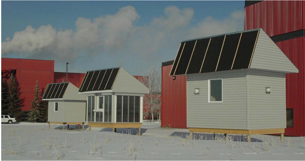
Figure 7: Experimental shelters used for the DHS solar system performance evaluation.
