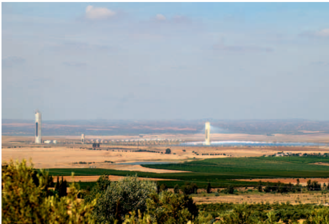
View of 3 CSP Power stations near Seville
