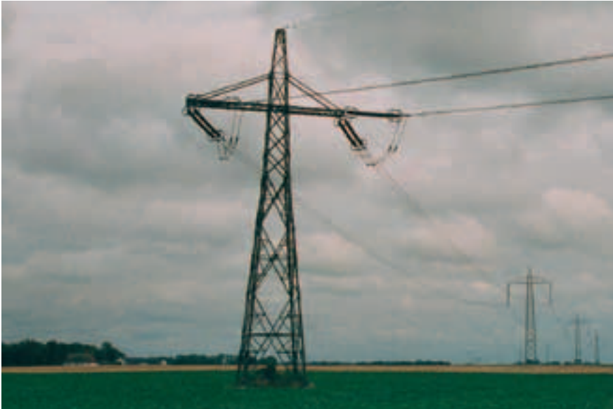
High voltage direct current (HVDC) cables in Sweden
