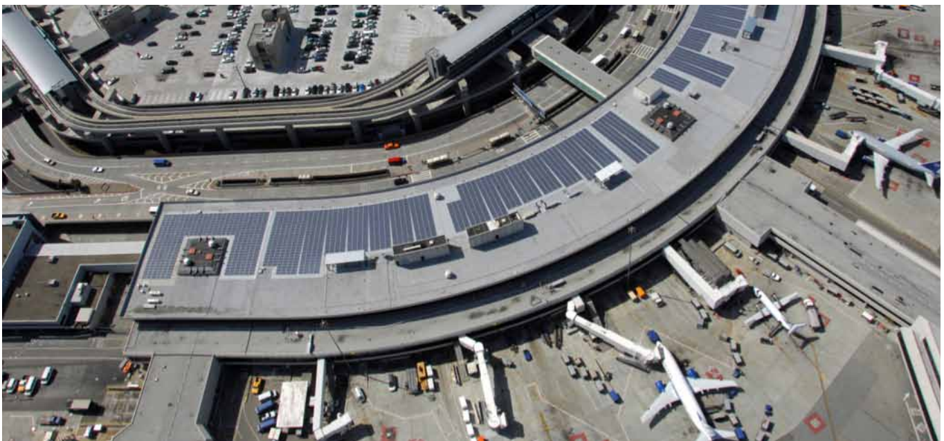
Below: Photovoltaic installation at San Francisco International Airport
