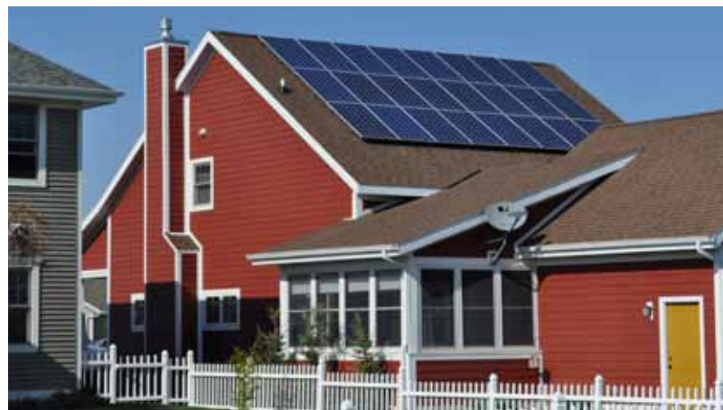
Residential photovoltaic installation in Plymouth, Wisconsin
