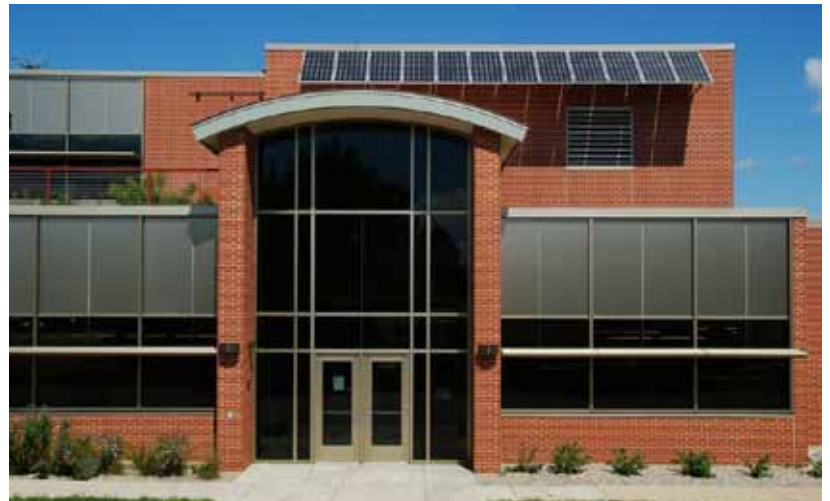
Photovoltaic installation on commercial building in Madison, Wisconsin
