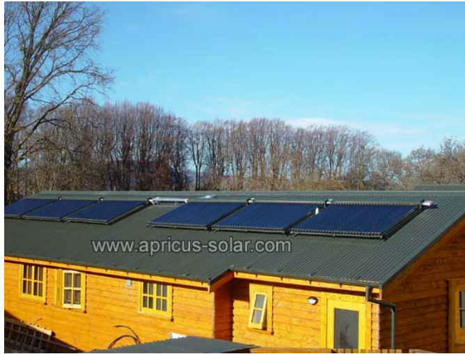
Apricus system installed by Sensible Heat Ltd. in 2004 on the guest cottages of the Wanaka Homestead in New Zealand.
