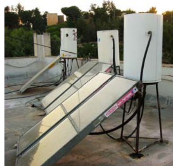
Example of a thermosiphon system, with solar collectors placed on the ground at a level below the house.
