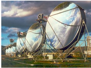
Parabolic dish technology, with Stirling engine to turn steam into electricity
