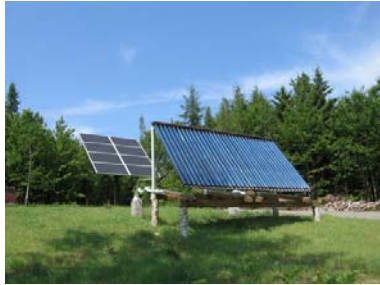
Example of a thermosiphon system, with solar collectors placed on the ground at a level below the house.
