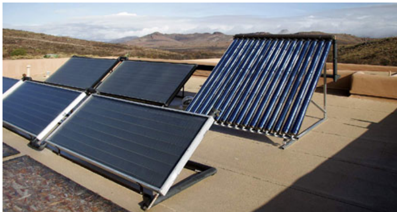
Two types of solar collectors: Flat panels (left) and evacuated tubes (right).
