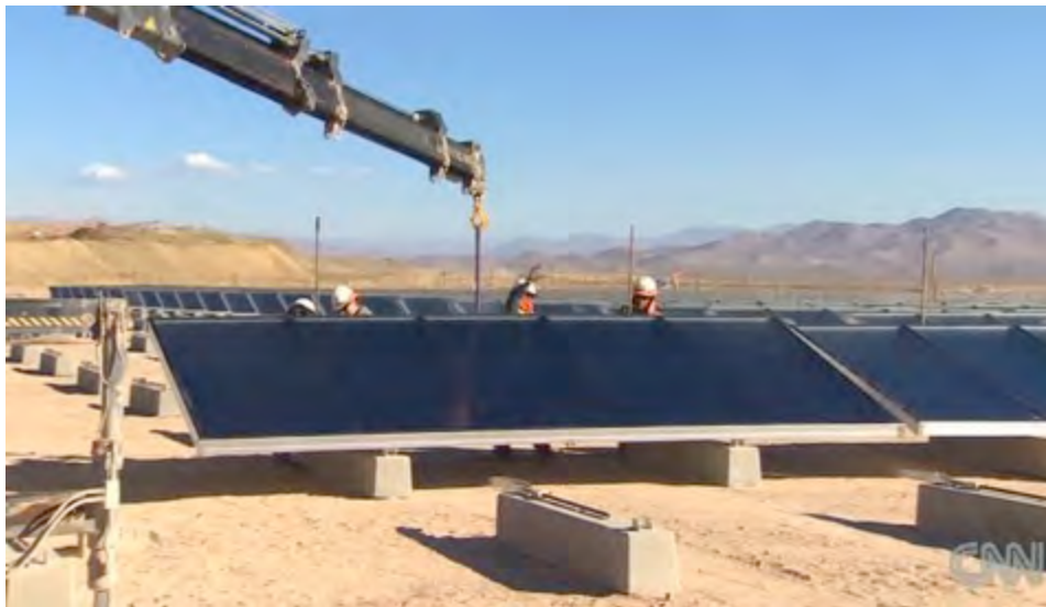
Figure 9: The world's largest solar thermal installation for industrial application at a copper mine in Chile 43
