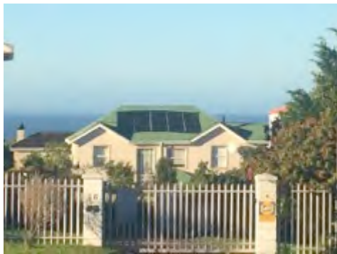
Figure 11: Typical rooftop installation of an unglazed swimming pool heater in South Africa
