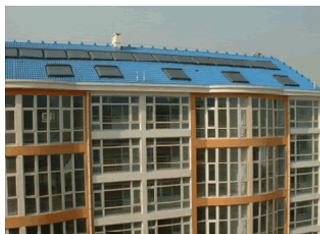
Fig. 5 Effect of solar collectors semi-imbedding into roofs of buildings [16]
