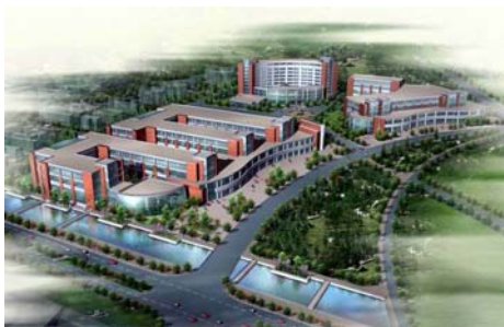
Fig. 19 The new solar lab of Shanghai Jiao Tong University
