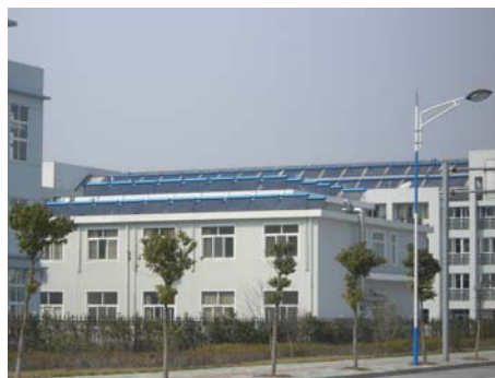
Fig. 18 The external appearance of the workers' eatery integrated with solar collectors
