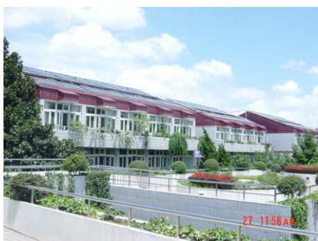
Fig. 3 Effect of solar collectors integrated into roof of building by overhead installation
