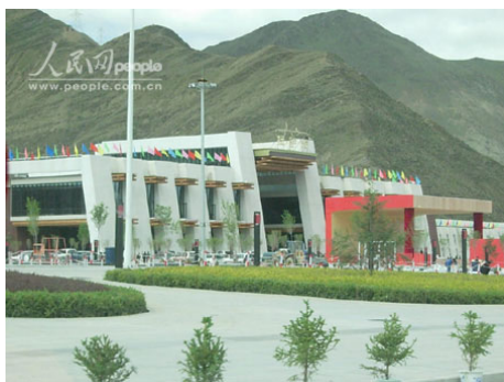
Fig. 2 Photo of Lasa railway station
