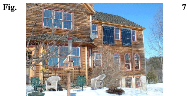
Fig. 7 Effect of solar collectors integrated into wall of building
