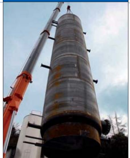
Fig. 2: Mounting one of the 55-m 3 solar storage tanks
