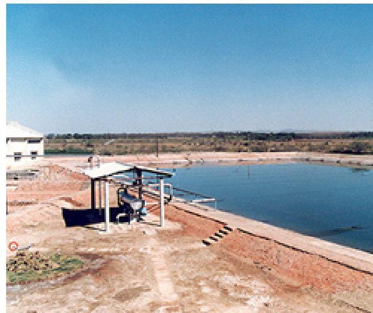
6000m 2 Solar pond at Bhuj dairy, Bhuj, Gujarat
