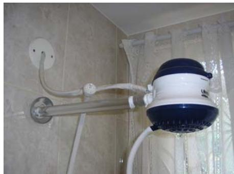
The graph of the average residential load curve in Figure 2 reveals that it is at peak-hour\_ normally between 06:00PM and 09:00PM\_ that the use of electric shower as a water heating device is the most widely spread [1].
