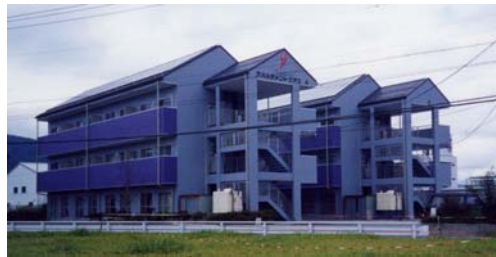
Solar apartment house (Chino City, Nagano Pref.)
