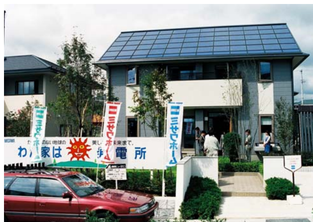
PV system with well insulated house and Solar DHW heating (Housing area near Akita City, Misawa Home Co.)
