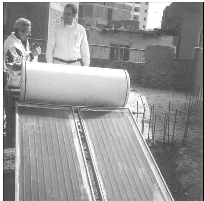
One of approximately 160 solar water heaters installed in urban and peri-urban areas (El Menia, Egypt).
