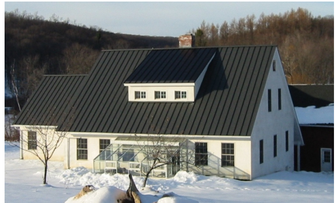
Fig. 1: The south side of the completed home with integrated solar systems.
