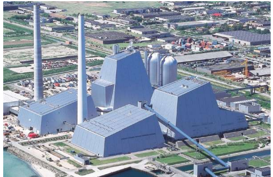
DONG Energy: Avedøre Combined Heat and Power Plant
