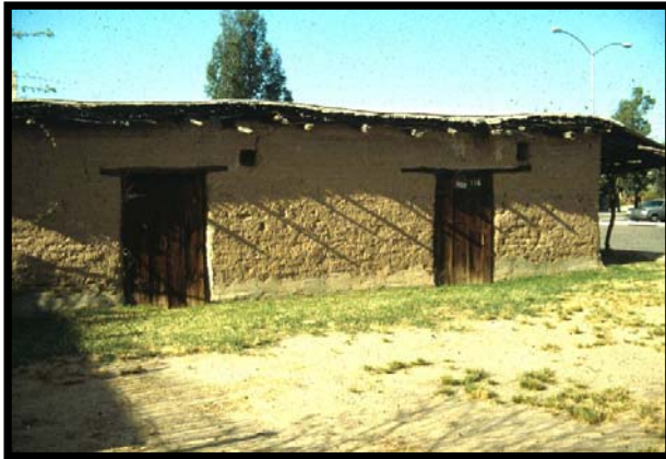
'South facing Trombe Wall of Storage Unit' (S B Kedare,ESE)
