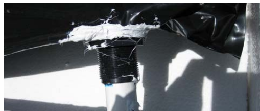
Figure 13: Caulk between bladder and fitting
