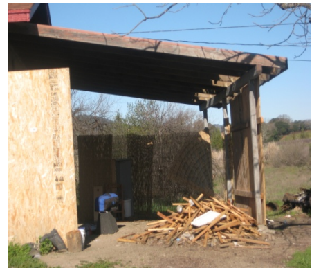
Figure 6: Potential installation site (not a very good one!)
