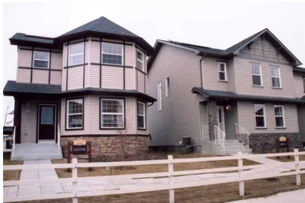
Sterling Homes built several different models of homes for prospective homeowners to choose from. Two of the model homes are pictured here. Photo by Sharon Boddy.
