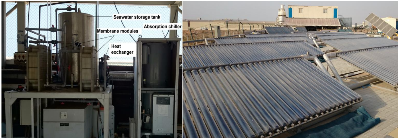
Figure 2. Solar thermal poly-generation unit
